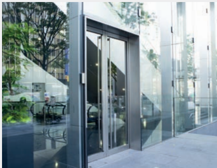
IP & ENTRANCE PANEL CAMERA MONITORING
