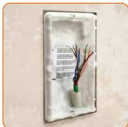
Removal of the existing entrance panel
